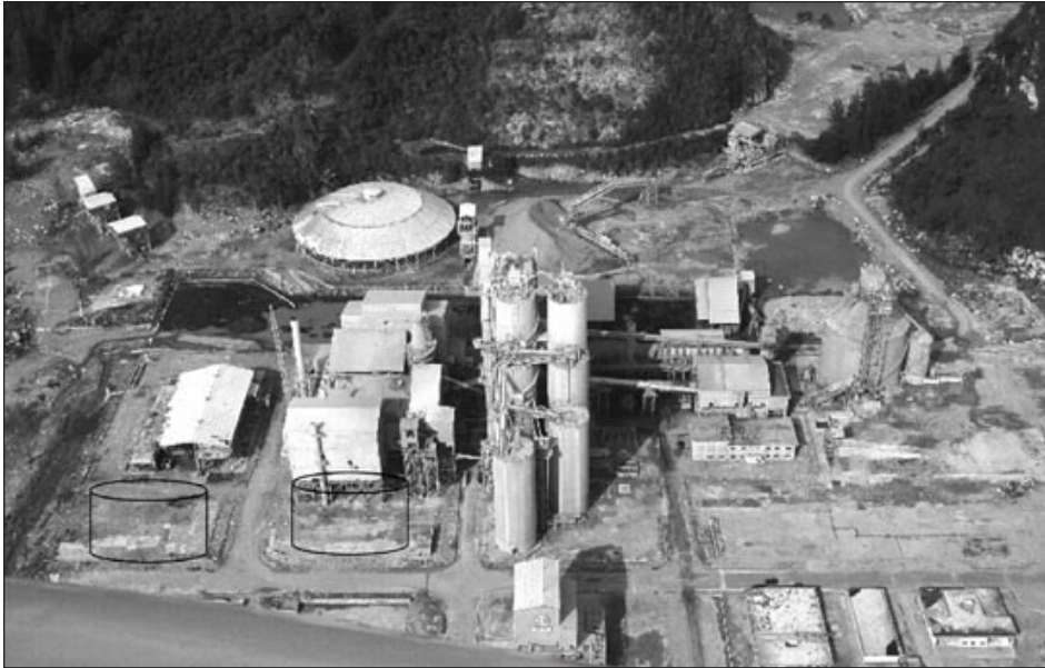
FIGURE 3 Aerial view of the La Farge Cement Plant. When the tsunami waves arrived, empty fuel tanks, indicated on the bottom left of the photo, became buoyant and destroyed small buildings to the right. The empty tanks also collided with the steel-reinforced cement silos but glanced off without damaging them.
