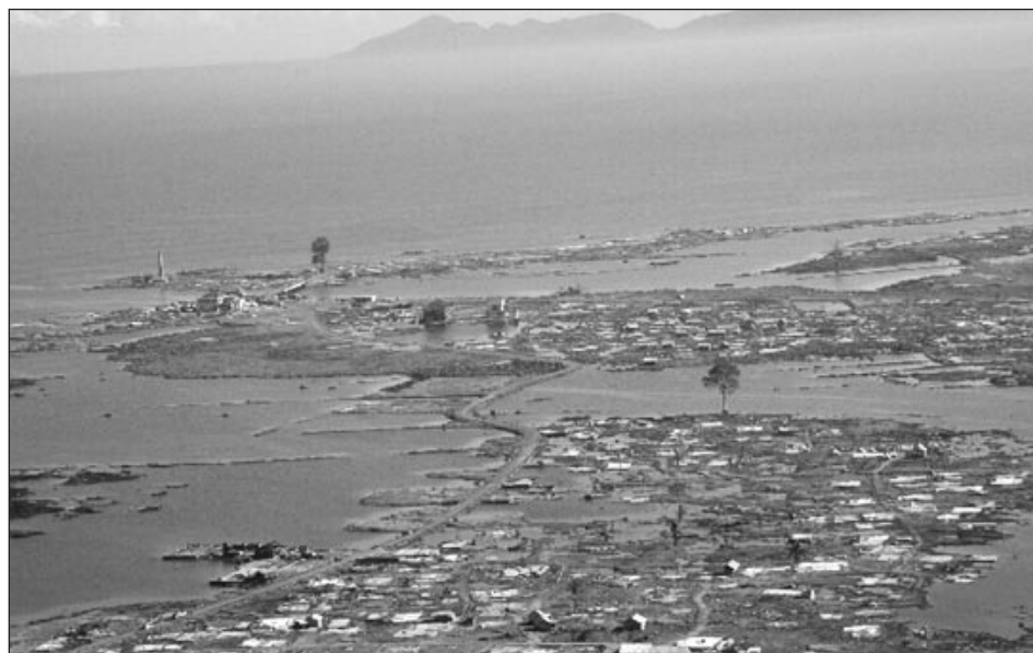
FIGURE 2 Aerial view of western Banda Aceh showing an area devastated by tsunami waves. Only concrete floor slabs of most houses remain.
