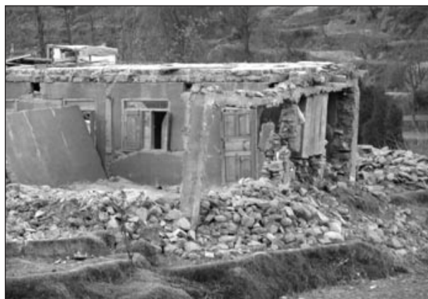
FIGURE 4 Collapsed building showing remains of a concrete bond beam.
