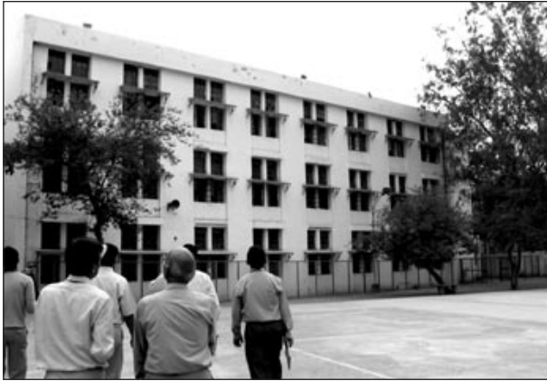
FIGURE 5 A school in Delhi, India, built of brick masonry scheduled for seismic rehabilitation.
